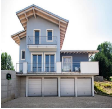
Figure 1: A pilot example of building to monitor
