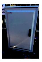
In the Open Fiber network the SFP usually is an outdoor cabinet with 20 splitters 1:16 inside. This is due to the needed flexibility to easily provide a dedicated GPON to at least 5 different OLOs. The cabinet is also engineered to host:
